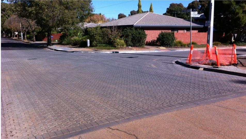
**Figure 1.** Permeable paving infiltrates stormwater into the road subgrade at the intersection of Kegworth and Wheaton Roads in Melrose Park, South Australia. As part of a broader treatment, this solution cost \$1M less than the alternative option of upgrading the pit and pipe network.
