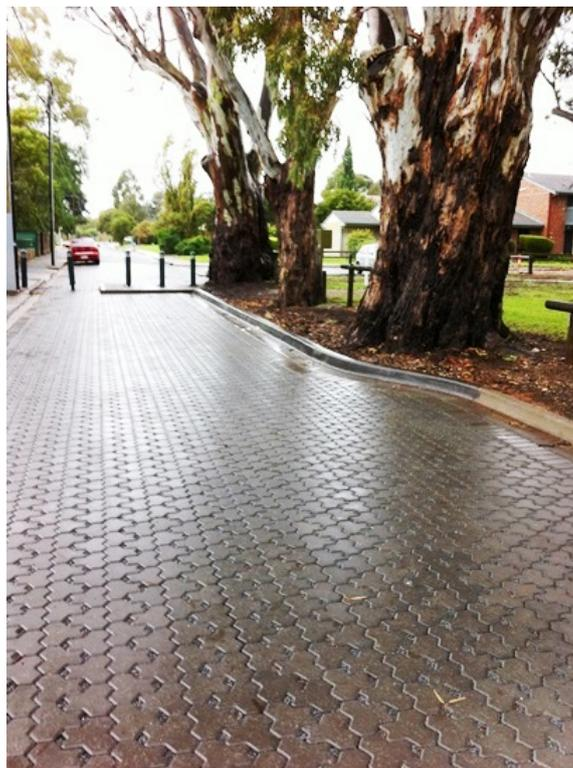
**Figure 2.** The absence of roots in road base material allowed its excavation without harm to nearby trees. Underdrains soak storm water from beneath the permeable pavement into the adjacent reserve as well as into the road subgrade; this has eliminated runoff from the paved surfaces.
