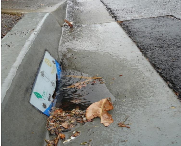
**Figure 9 - Functioning Inlet at City of Mitcham Council**
