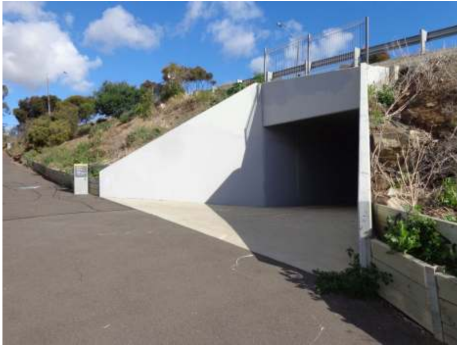
Figure 2. An expensive retrofitted tunnel providing access under a busy suburban road for non-vehicular users. The tunnel addressed major user safety concerns, but at very high cost.
