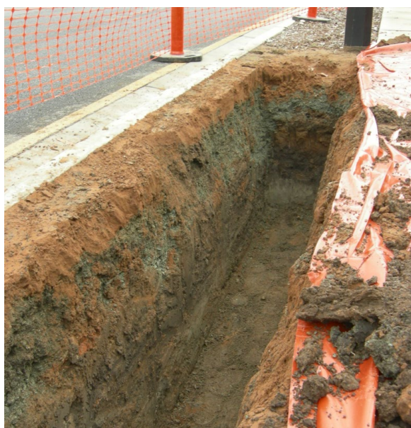
Figure 17. The tree soil trench provided a pathway for roots to access natural site soil beneath a layer of compacted road base material (image: C Lawry).
