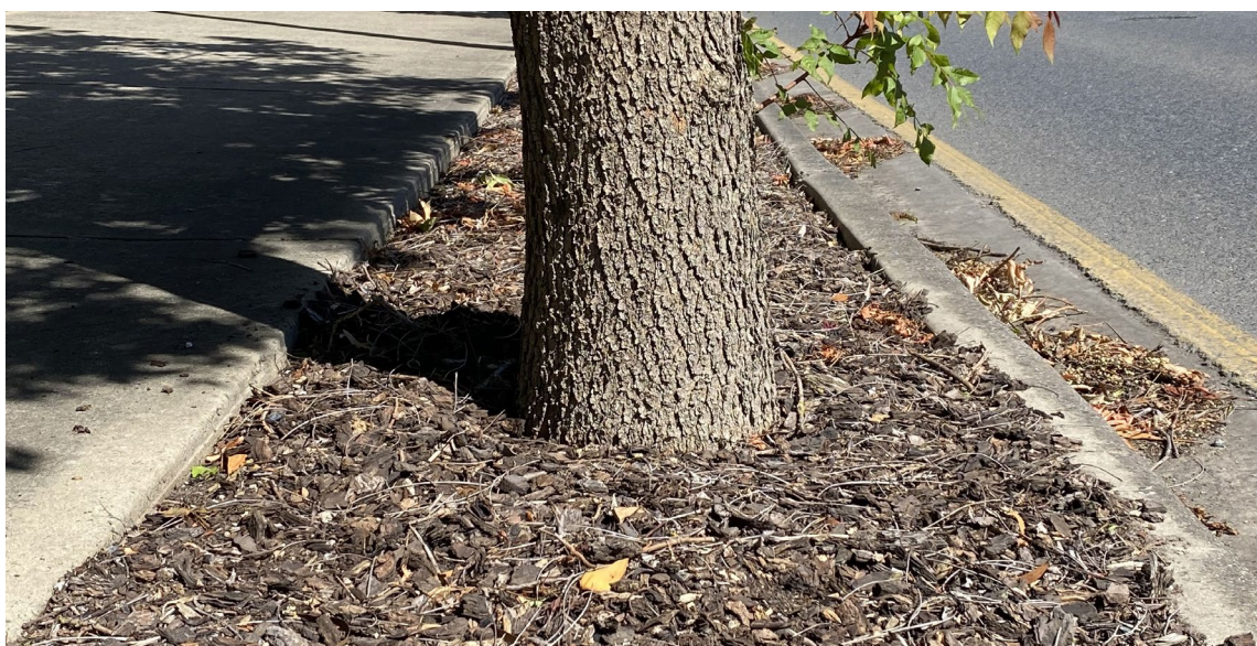
Figure 19. Chinese pistachios well-established in 0.6 m wide tree trenches showed no impact after 13 years on nearby kerb, road or path assets (image: T Johnson 2023).
