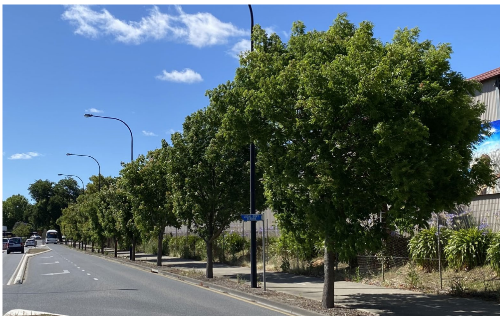
Figure 18. Chinese pistachio established consistently in tree trenches excavated to 1.4m deep between the kerb and shared-use path (image: T Johnson 2023).
