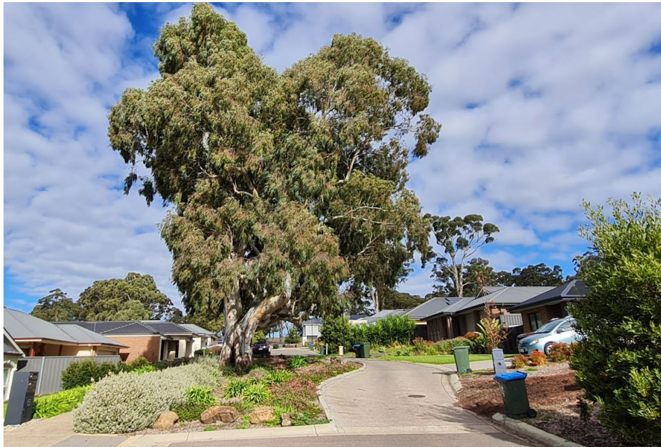
Figure 11. Novel alignment of driveway links and use of concrete road and ballast base over uncompacted subgrade protected the root zone to preserve a Blue gum ( E. leucoxylon )(top) and River red gum ( E. camaldulensis ) in Bremer Street (photographs: C Lawry).
