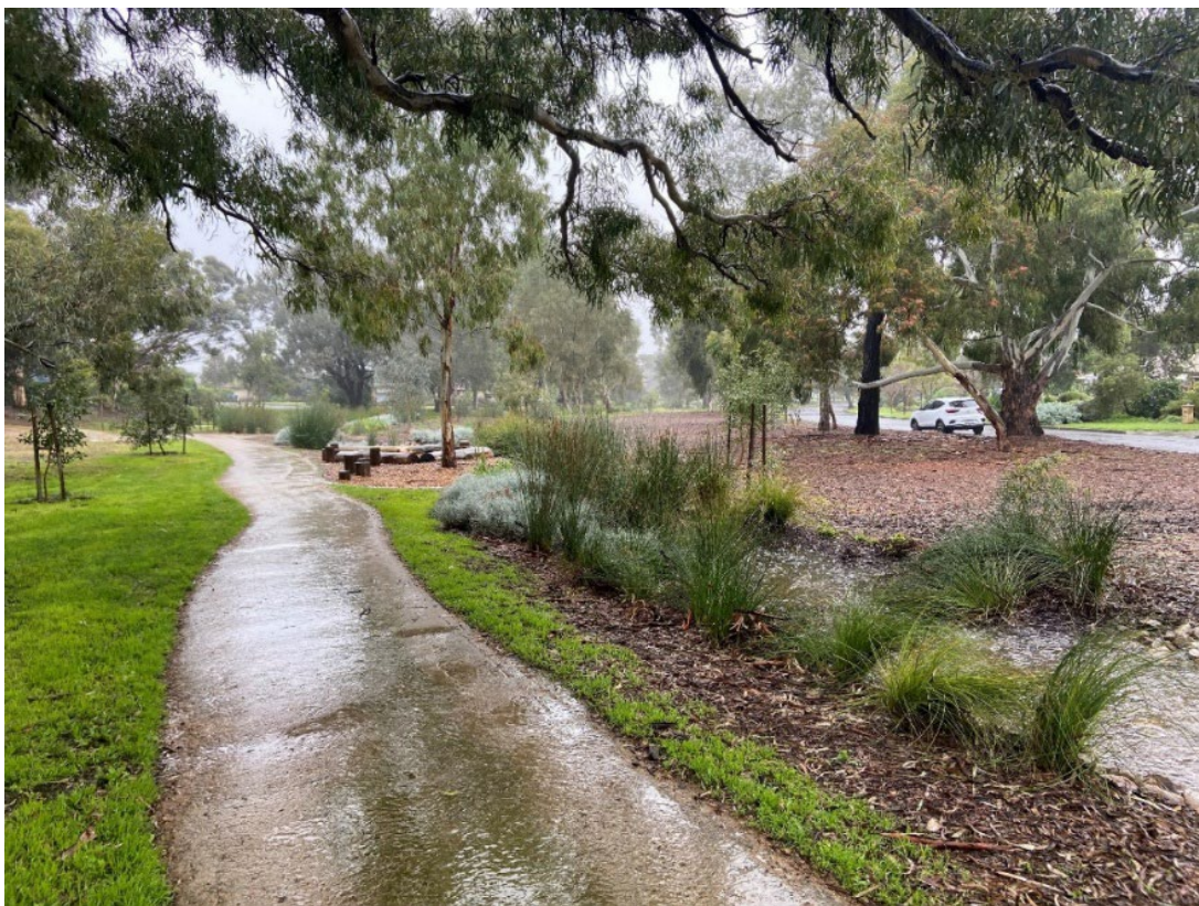
Figure 4. Pasadena Biodiversity Corridor post-construction showing the daylit creek
