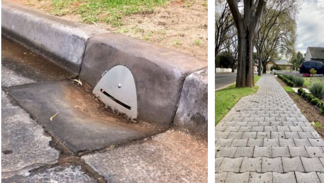
Figure 6: Kerb inlet and permeable footpath installed in the City of Mitcham
