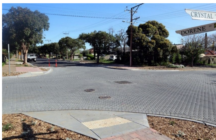
Figure 1: Permeable paved intersection supporting garden beds with subsurface passive infiltration
